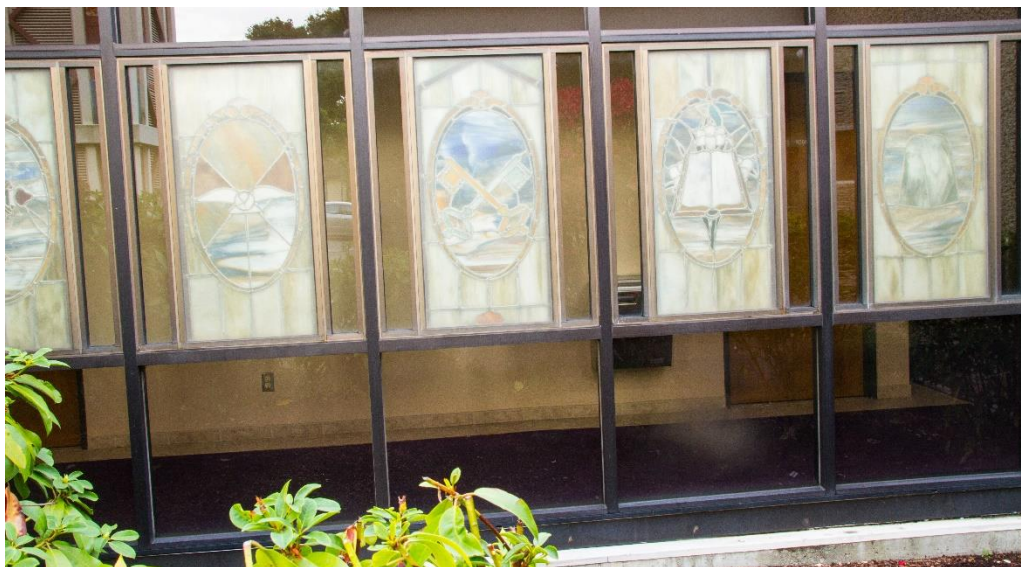
Outside View of Windows leading into the CHAPEL.
