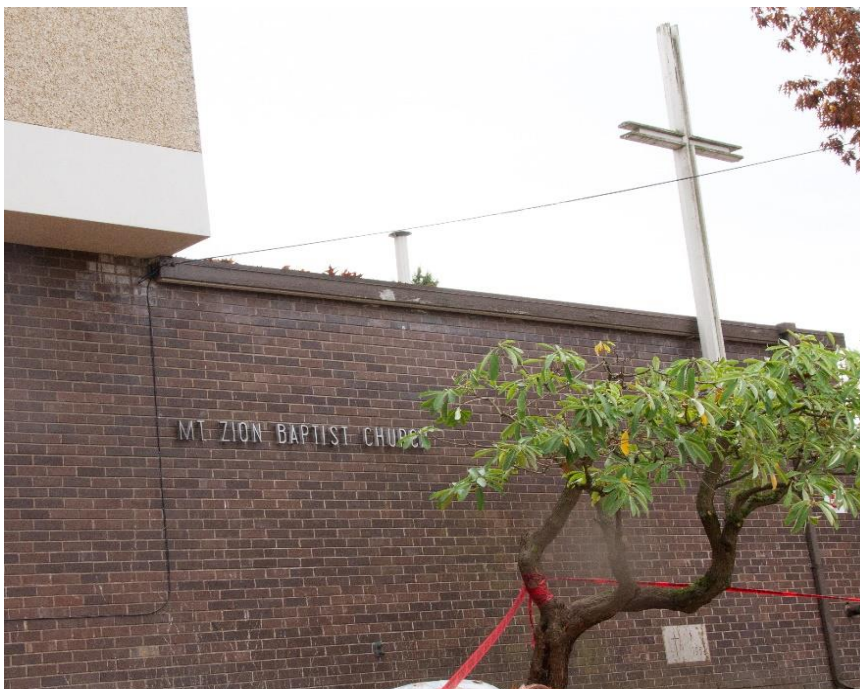
View of Educational Unit on East side of Church.
