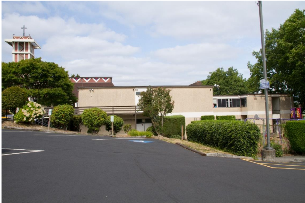
Views from Southside of Church including parking lot.
