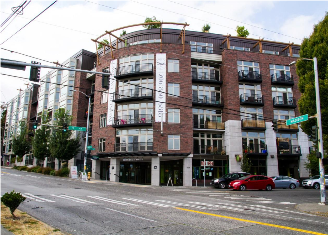
Photo of Area Surrounding the Church.
