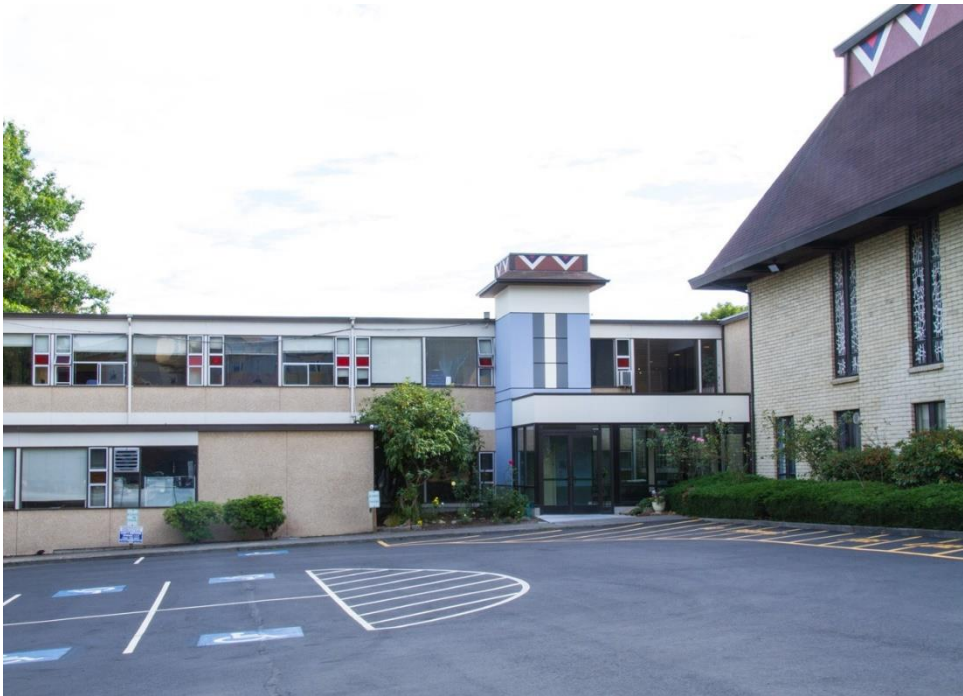
View from North Entrance into the Church from Parking Lot.
